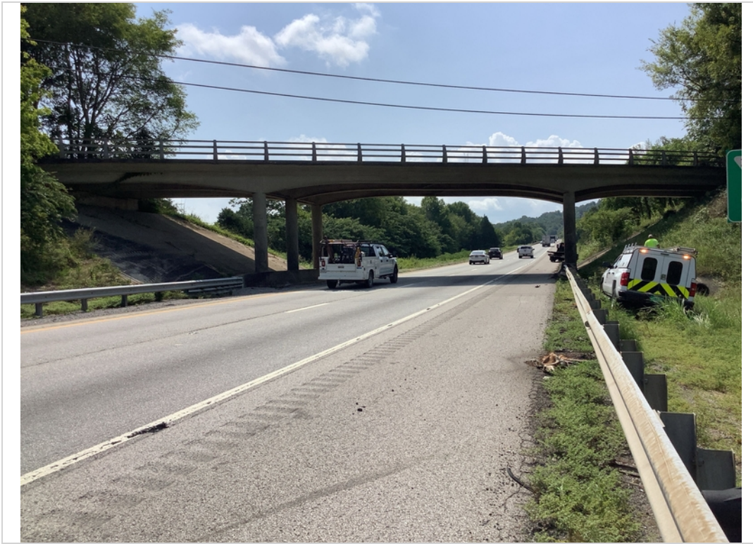
Underclearance looking ahead on underpass route
