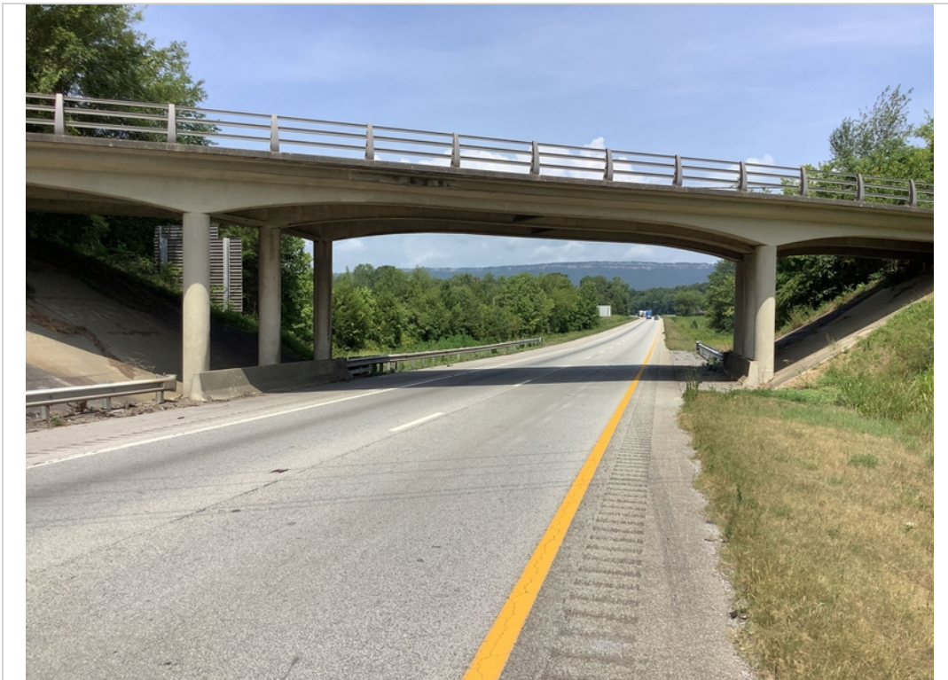
Underclearance looking back on underpass route
