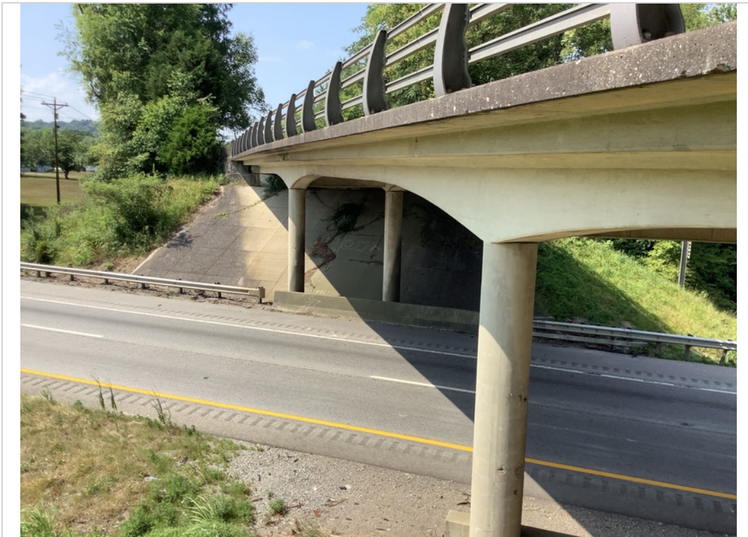
Left side view of structure
